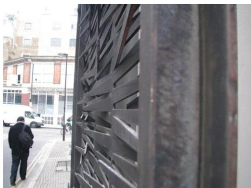
Working Metals has always embraced the challenge presented by its creative customer base and has produced some stunning results using the new Metallisation MK61 Flamespray equipment. Amin Taha Architects, one of Working Metals customers, recently specified thermal sprayed bronze to be applied to steel
