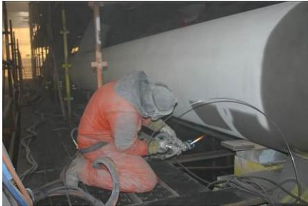
Metallisation customer, Gardwell Coatings Limited, based in East Anglia, has applied Thermal Sprayed Aluminium (TSA) to an offshore oil platform to protect the structure from corrosion, using Metallisation MK73 flame spray equipment.
