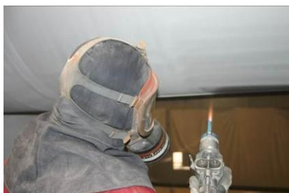
the job at any one time and sprayed an average of around 100 square metres of TSA a day. Given the complexity of the job, which included the internal coating of the 1m diameter tubular sections, this production rate is quite an achievement.
