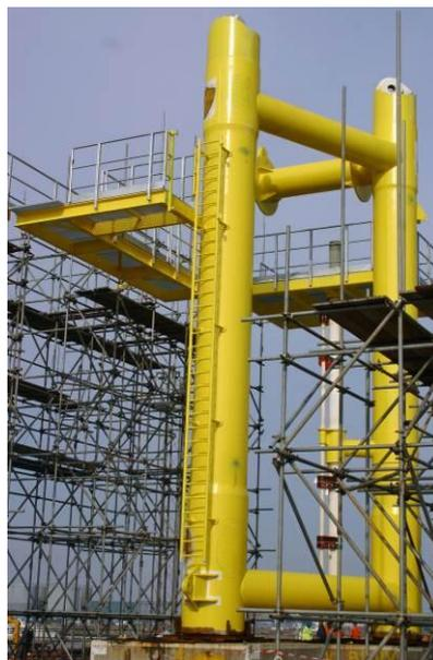
Gardwell Coatings completed the metal spraying process on site at the SLP Engineering site in Lowestoft using the Metallisation MK73 system. Gardwell Coatings recently purchased an additional three MK73 systems with long supplies packs. With
