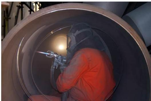
Around two thirds of the external surface of the columns, which will be in the splash zone and exposed to the harsh North Sea, were TSA'd to the same thickness, sealed with epoxy sealer and top coated with a PU topcoat. In addition, a number of stainless steel parts and riser pipes have also been TSA'd and sealed. In total, around 450 square metres of the centre core has been TSA'd.
