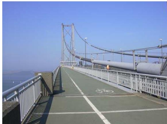
structure, which makes up the bridge, to protect it from corrosion. The contract to protect the bridge was split between Metallisation and Merseyside Metal Sprayers Ltd. The latter company was commissioned to treat the 1200 balustrades and vehicle grillage panels.
