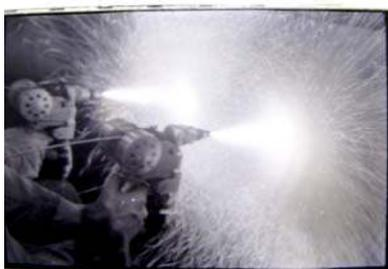
Each of these giant sections was then treated individually, starting with the cleaning process using grit blasting. Grit blasting is the most effective way to remove scale and rust from steel to provide a clean, prepared surface for the zinc to adhere to. The second stage was to spray the steel surface with zinc
