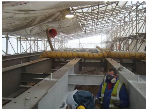
the timber deck, the steel structure was covered with a large industrial shrink wrap enclosure, under which all of the thermal spraying took place. The tent was fitted with an extraction system, de-humidifiers and heaters to create the optimum environment for surface preparation, metal spraying and painting of the bridge. The enclosure also ensured that dust generated during the surface preparation and coating process was contained and didn’t contaminate the local environment.
