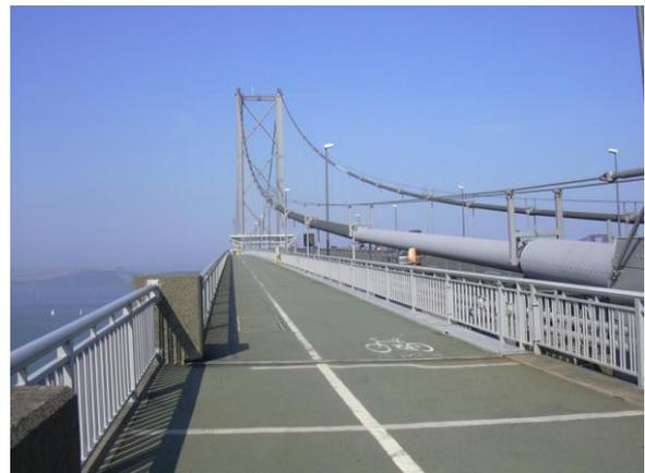
contract to protect the bridge was split between Metallisation and Merseyside Metal Sprayers Ltd. The latter company was commissioned to treat the 1200 balustrades and vehicle grillage panels.
