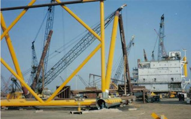
As well as inland applications, APS has used Metallisation equipment to spray offshore installations. Various oil and gas platform structures have benefited from the application of thermal sprayed aluminium (TSA).
