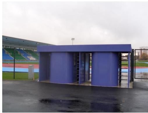
The second project was to protect the entrance turnstiles at a defence site in the UK. Again strong, robust, hardwearing surface protection was required, which has been delivered by metal spraying the turnstiles with zinc. This time Electro Metal Depositors has provided a 20 year guarantee to its client.
