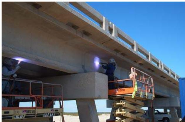
good key to enable the coating to bond. The coating would then be applied with either a Metallisation Arc140, Arc701 or Arc170 system, depending on the size and accessibility of the structure. Historically on installations in the USA, typical bond strength is in the region of 1 to 3MPa for zinc and coating thickness would be between 300 and 500 microns.
