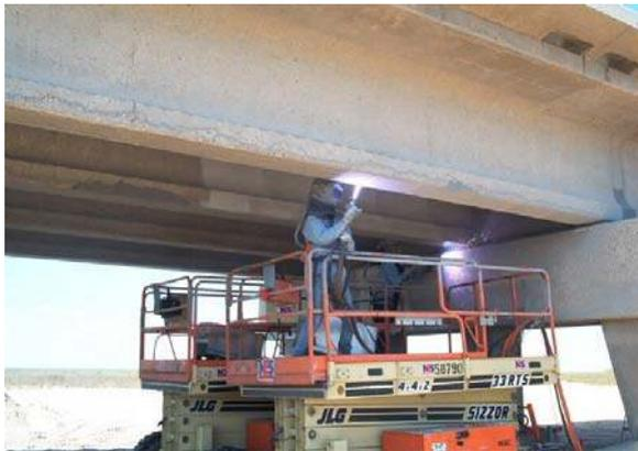
Another significant application of the Al-Zn-In alloy in the US is the San Luis Pass Bridge near Galveston, Texas. More than 30,000 m<sup>2</sup> of concrete beams and caps are protected with this alloy, installed using Metallisation ARC 700 units by Corrosion Restoration Technologies of Jupiter, Florida.
