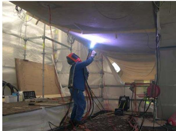
solution. The precast concrete panels, which are 2.6 x 2.8m of lightly reinforced 8cm thick units, form the underside of the concrete viaducts carrying road traffic to and from a busy terminal complex. Run-off from de-icing salt has led to an important level of chloride in the panel concrete. Although the panels are not structurally significant, spalling could present a hazard to passing traffic.
