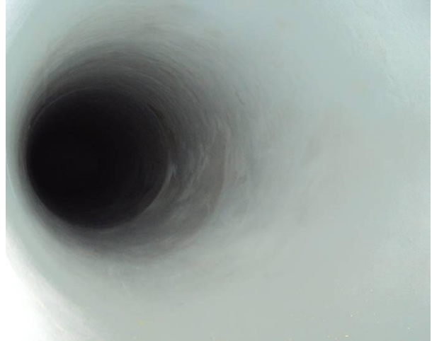
Figure 2: Pipe surface after metal spraying
